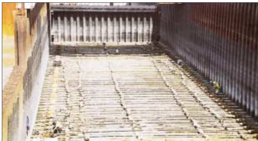
Cardiff Bay Barrage
